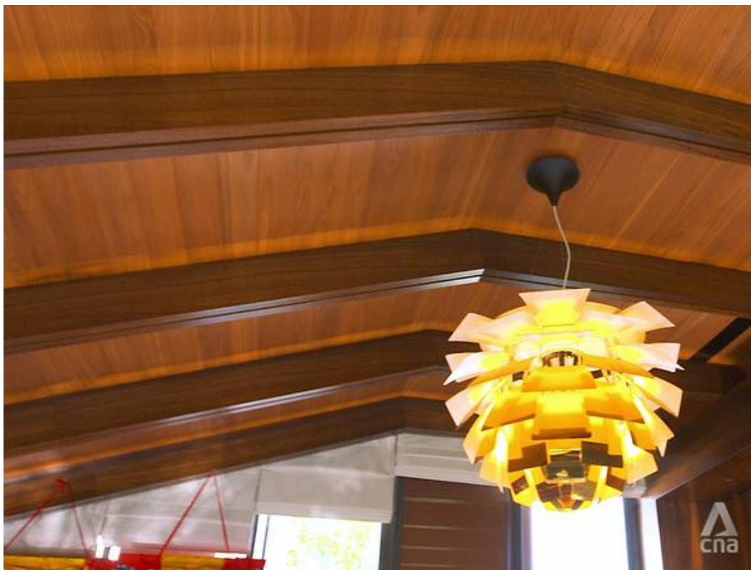
The roof was restored to its former glory. (Photo: Threesixzero Productions)
