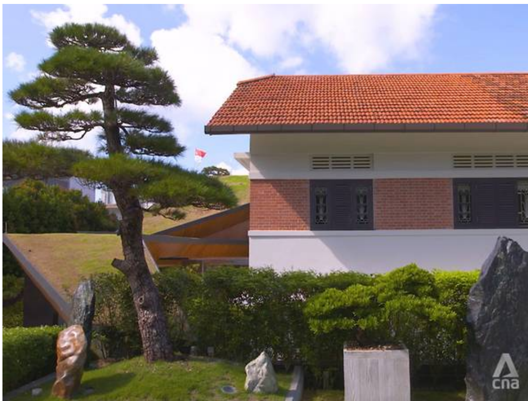
The colonial bungalow is nearly a century old, and has conservation status. (Photo: Threesixzero Productions)
